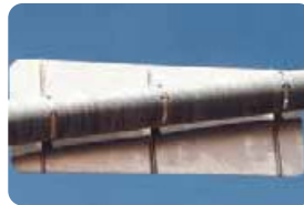
Mast Arm Sign Installation
