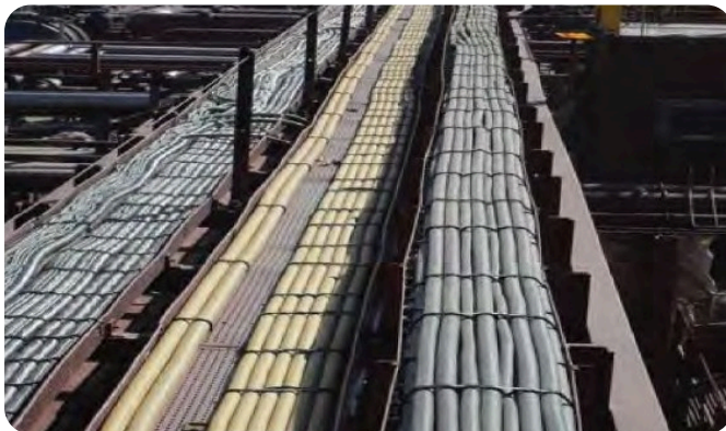
Cable management: reduces the risk of cutting or abrading cable
