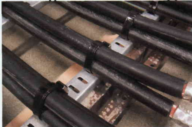
Fig 2; Double wrapped AE455 band / LE155 Clip positioning
