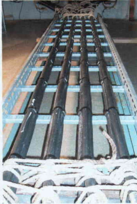
Fig 1; Test rig fitted with 4 parallel trefoil cable runs
